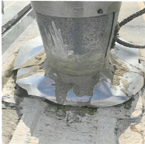
Remove previous repair and install new dektite boot
